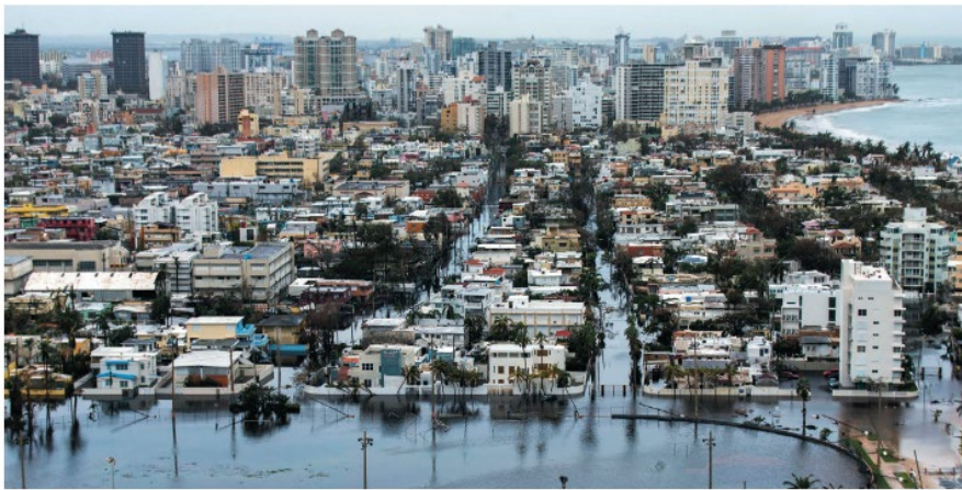
The coastal city of San Juan in Puerto Rico was flooded after Hurricane Maria hit in September 2017.
