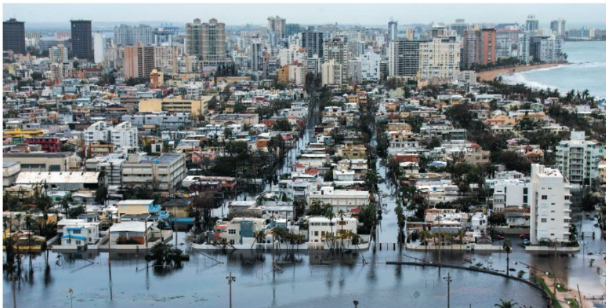
The coastal city of San Juan in Puerto Rico was flooded after Hurricane Maria hit in September 2017.
